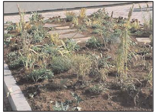
A semi-extensive garden on Toronto's City Hall roof (source: www.peck.ca/grhcc/overviewdemo.htm )
